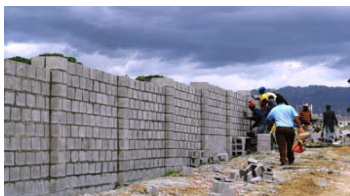
The boundary wall
